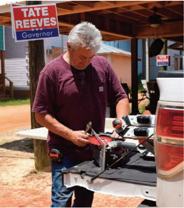
Kevin Alford does some construction on Cabin 215.
